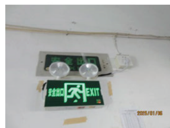
10-Safety exit sign combined emergency light.JPG
