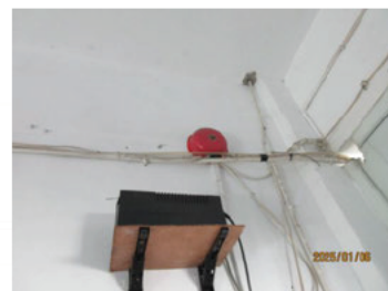
14-Fire alarm with backup source.JPG
